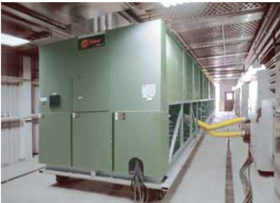
Air-cooled Run Test Facility shown with an RTAC 500 ton unit
